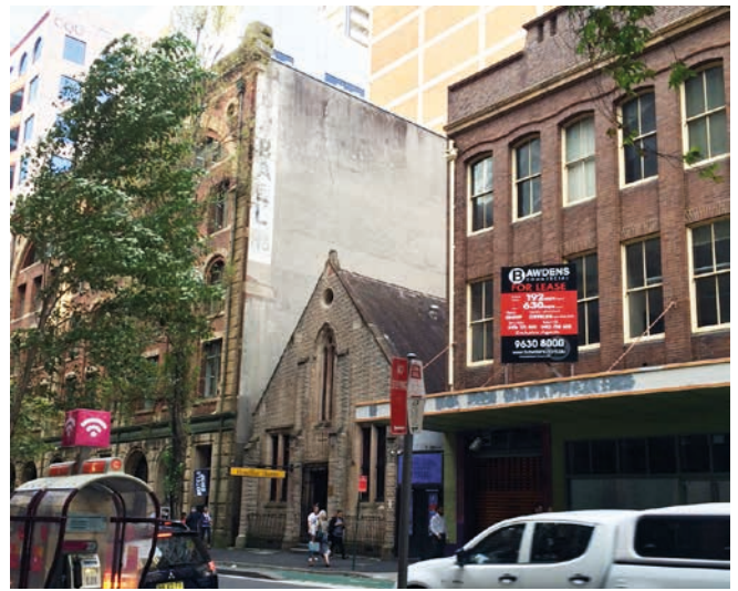
E_32 York Street SCA - Kent Street 420 Kent St Heritage Item
